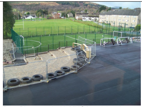
Rear Playground with MUGA and tiered seating area
