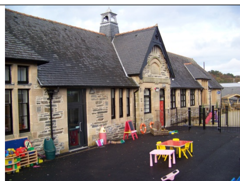
1881 Building - Elevation from Park Road
