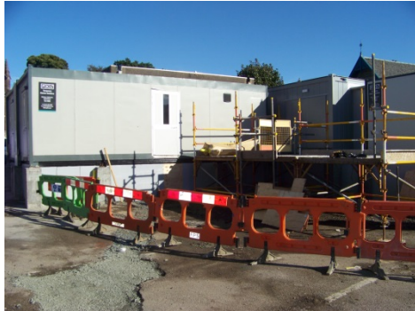
Modular Kitchen Installation
