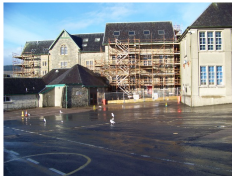
Scaffolding to West Wing
