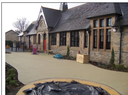
1881 Building - Elevation from Park Road
